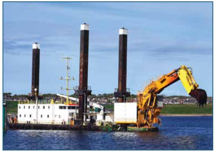
Backhoe Dredge, © Alan Smillie/Adobe Stock
